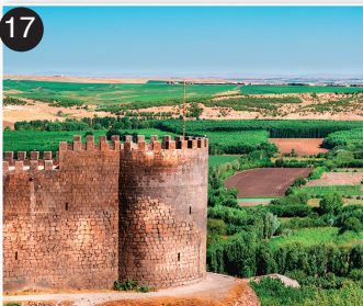
Diyarbakır Fortress and Hevsel Gardens Cultural Landscape (2015)
